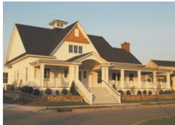
Public spaces are an important part of a traditional neighborhood design. DPA designed the Community Center, shown here, as well as many of the model production homes.
